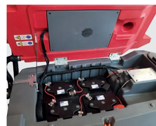
Compartment des batteries
